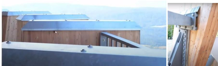
**Figure 1.** a; metal caps for columns, b; dropper detail (Aklan, 2021)
