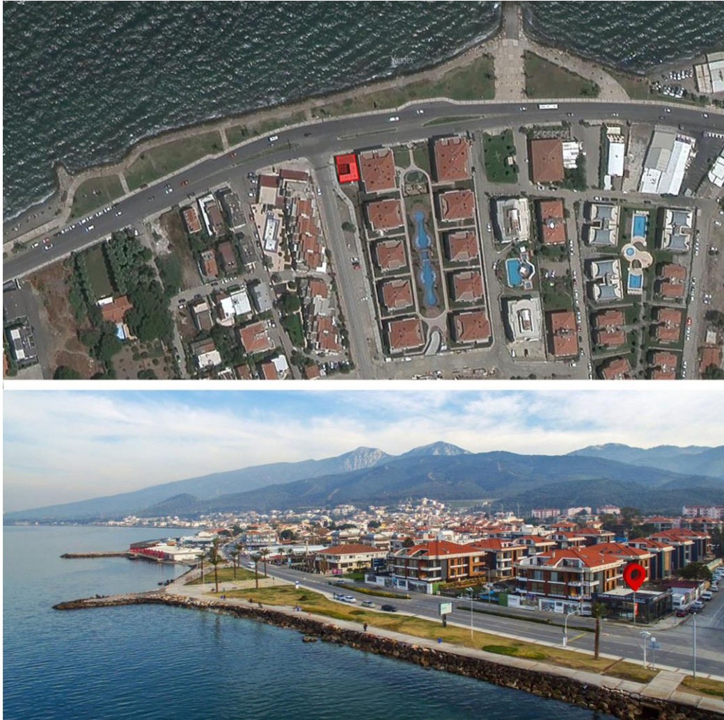
Figure 1 - Project site [Above: Satellite view; Below: Aerial view] (Photo credits: Çiçek Kardeşler İnşaat Ltd. Şti.)
