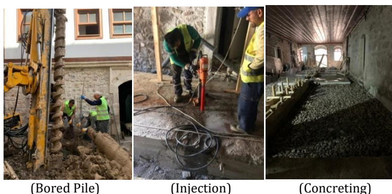
Figure 17. Ground reinforcement in 2020 (Ankara Directorate for Surveying and Monuments, 2021).
