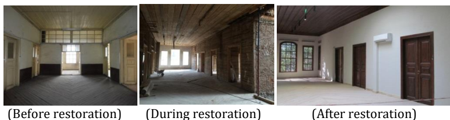
Figure 13. Restoration works (General Directorate for Cultural Heritage and Museums, 2021).
