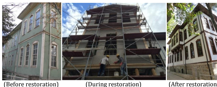
Figure 14. Restoration works (Ankara Directorate for Surveying and Monuments, 2021).
