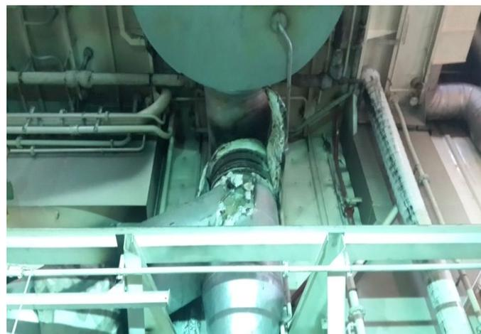
**Figure 5.** The funnel loop some parts of which fell of and uncovered for repairs
