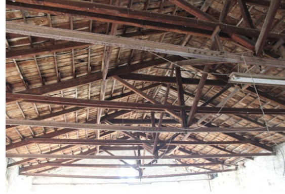
Fig. 14. Roof Construction of the Soap Factory Building (Photographed by Interior Architect Elif Türkmen)
