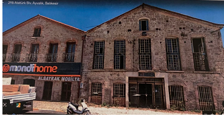
Fig. 19a. North Facade View of the Soap Factory and its Twin Building 43
