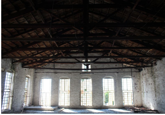
Fig. 13. First Floor and Windows of Soap Factory Building (Photographed by Interior Architect Elif Türkmen)
