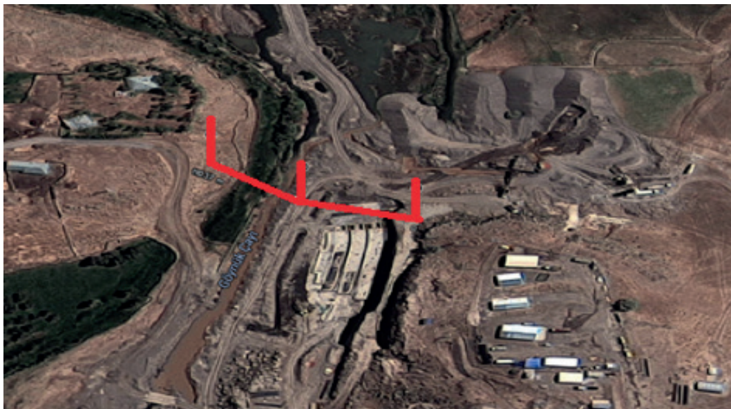
Figure 26. Dam-type reservoir for Saf HPP
