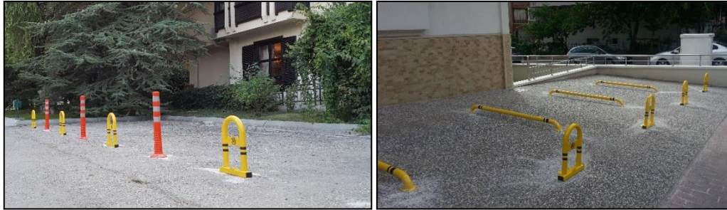
Figure 8. Fixed barrier types used between manual personal barriers.
