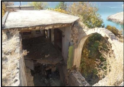
**Figure 31.** The soil roof torn down
