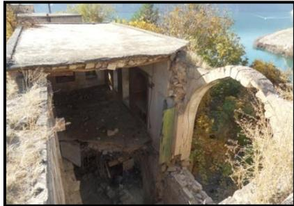
**Figure 31.** The soil roof torn down
