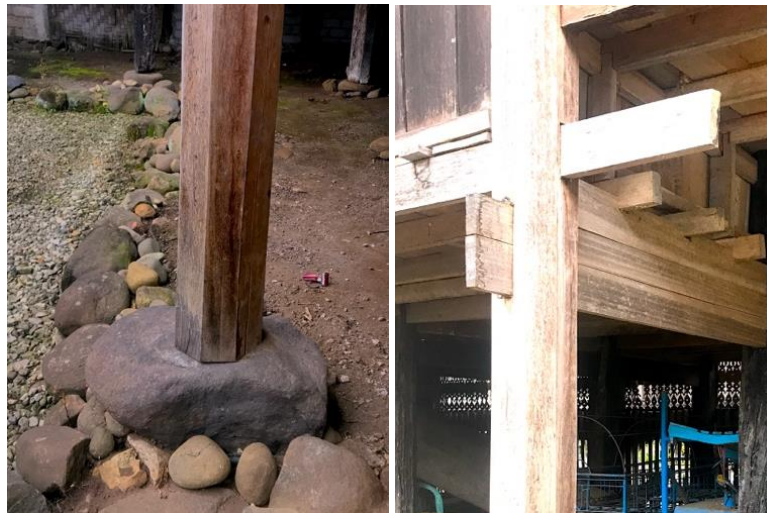
Figure 4. (left) The stone base (sandhi) (Johanita Anggia Rini, 2020)
