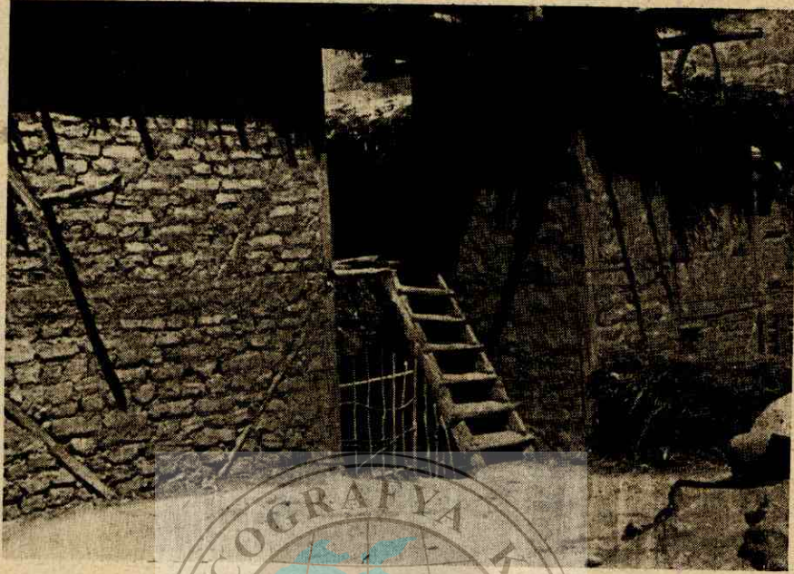
Orta Sakarya vadisinde kerpiçle inşa edilmiş yeni bir ev tipi. A new two-storeyed house type. It is made of with sun-dried bricks and thin woods.
