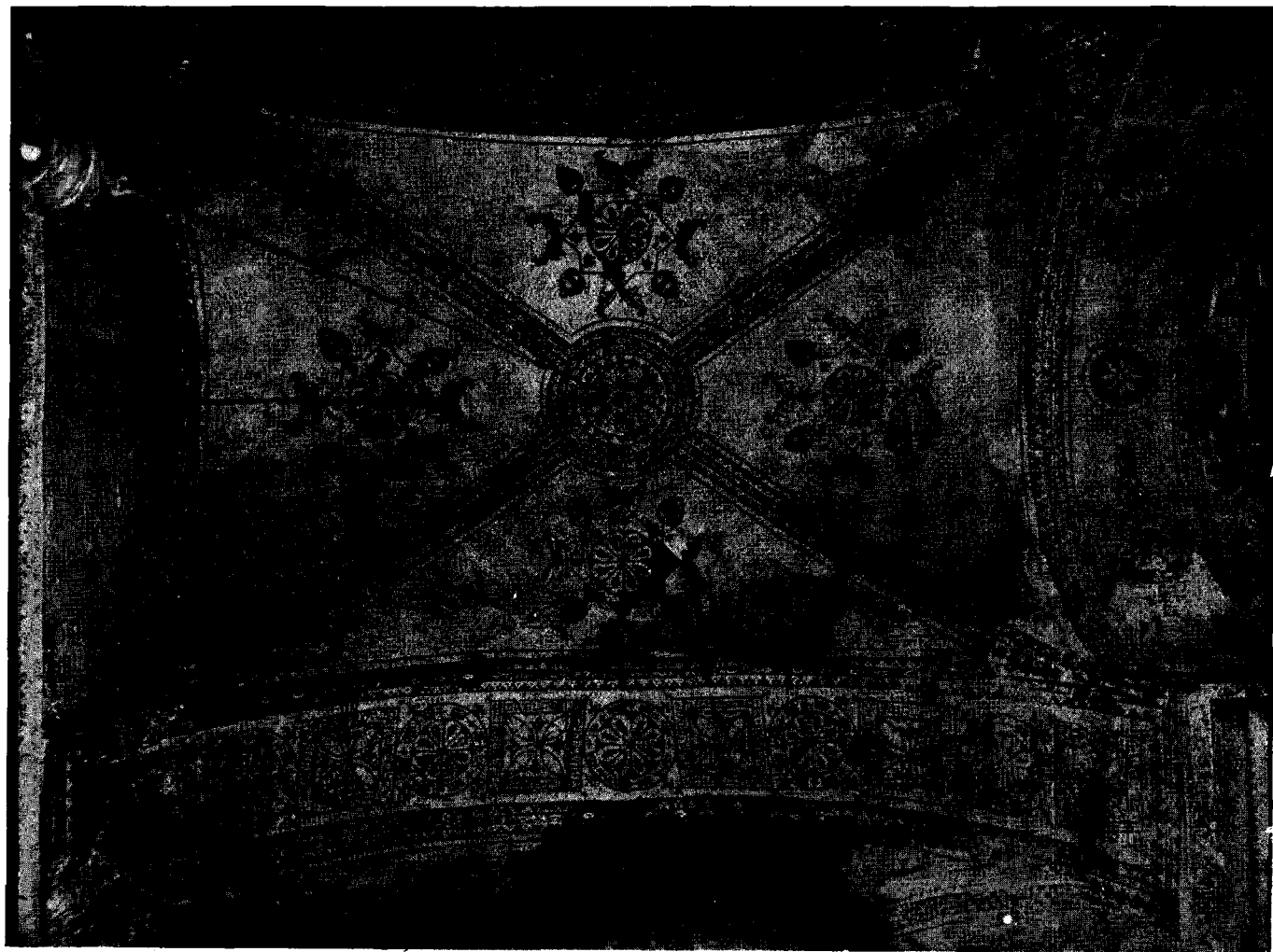
Golden ceiling of the Narthex, now cleaned.
