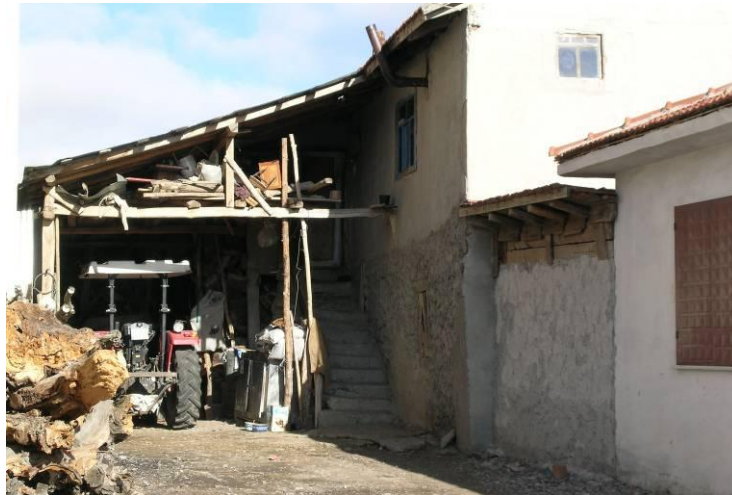
Figure 17. Repaired timber-framed building
