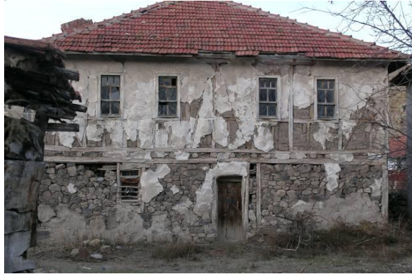
Figure 7. Composite structure: Stone masonry first floor and timber-frame with sun-dried brick infill (Yuva Village).
