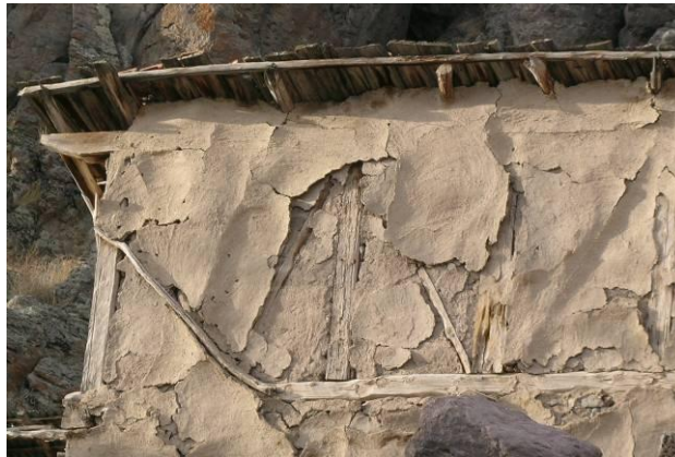
Figure 4. Diagonal members of a timber-framed building
