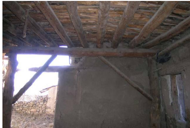
Figure 10. Posts, beams and girders (House 1).
