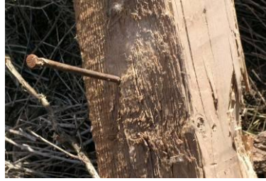
Figure 13. Nail used to tie the timber elements
