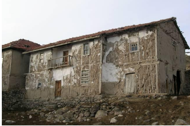
Figure 6. Timber-framed structure with sun-dried brick infill (Yuva Village).
