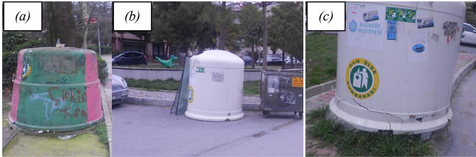
**Figure 3.** Images of some waste glass bins in bad situations (a): worn as unsuitable to use (b): threatening traffic safety (c): threatening health
