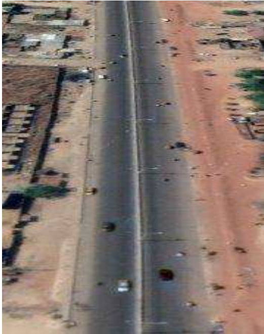
Figure 1: Aerial view of Gwarzo road
