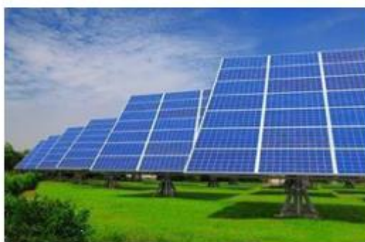
Start of the construction of the solar PV
