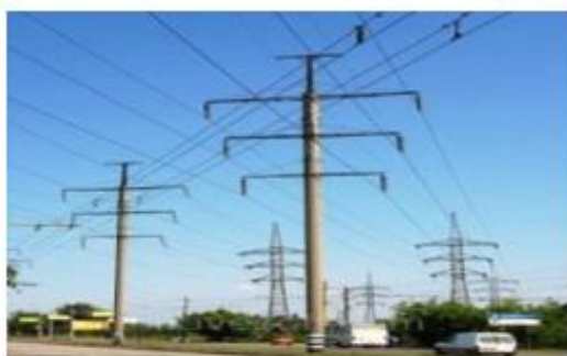
Start of the construction of the connection line
